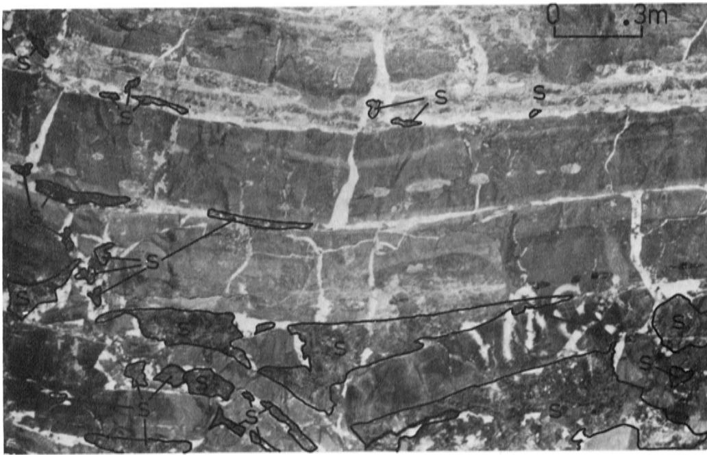
Figure 12. Photograph showing partial collapse of hanging-wall dolostone above a dissolution-collapse breccia in the Elmwood mine, stope 15-78 #3. Open spaces in breccia, gash veins, and bedding partings are filled with calcite (white) and sphalerite (s; dark grey).
